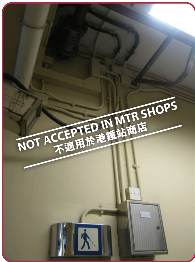
General Conduits - UPVC or PVC (not accepted in MTR station shops) 一般導管 — 硬塑膠料或聚氯乙烯 (不適用於港鐵站商店)
